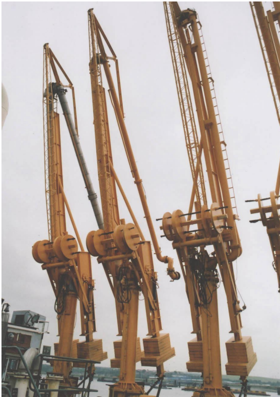
Figure 8 - typical loading arms without vapour return facility
